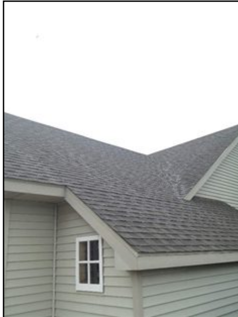
1. Asphalt shingles
