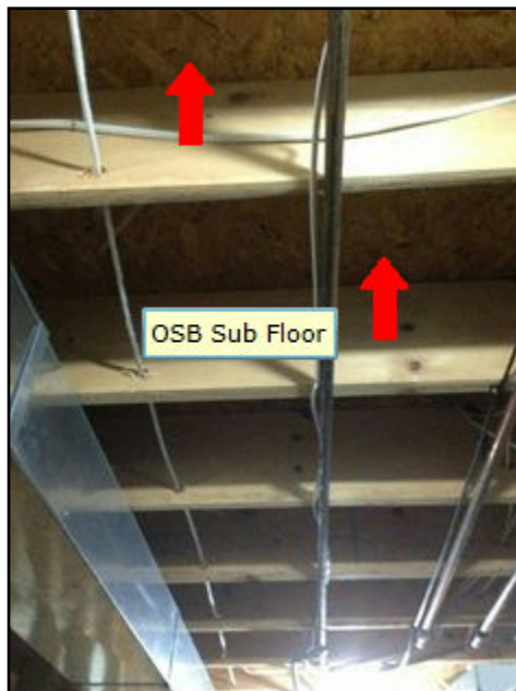
17. Sub floor - OSB (Oriented Strand Board)
