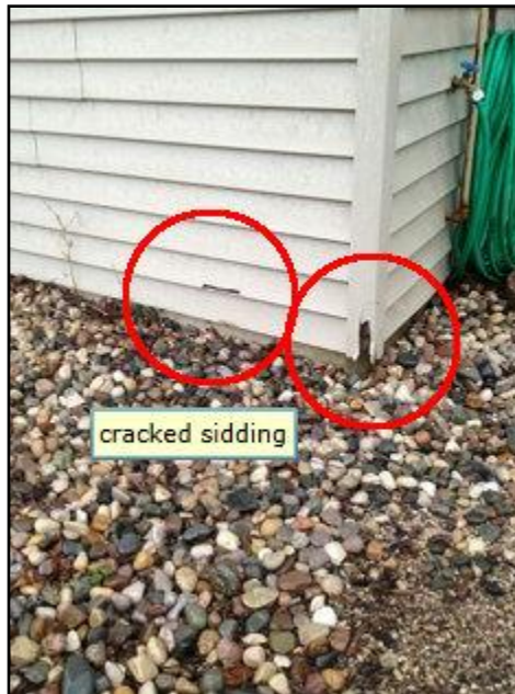
13. Mechanical damage
